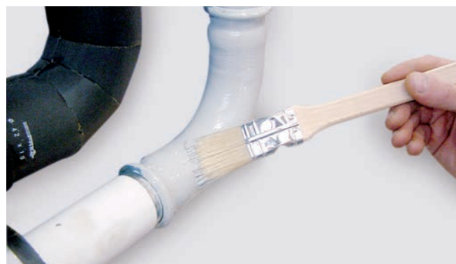
Figure 42 – Varnish of the connections and pipes with primer.
