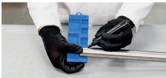
Figure 30 - Marking the insertion depth
