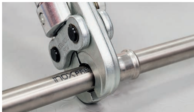
Figure 37 – Making the press connection
