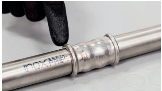
Figure 38 - Checking the press connection
