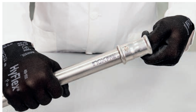
Figure 36 – Inserting pipe into the press fitting
