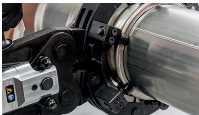
Figure 40 – Press assembly phase 2
