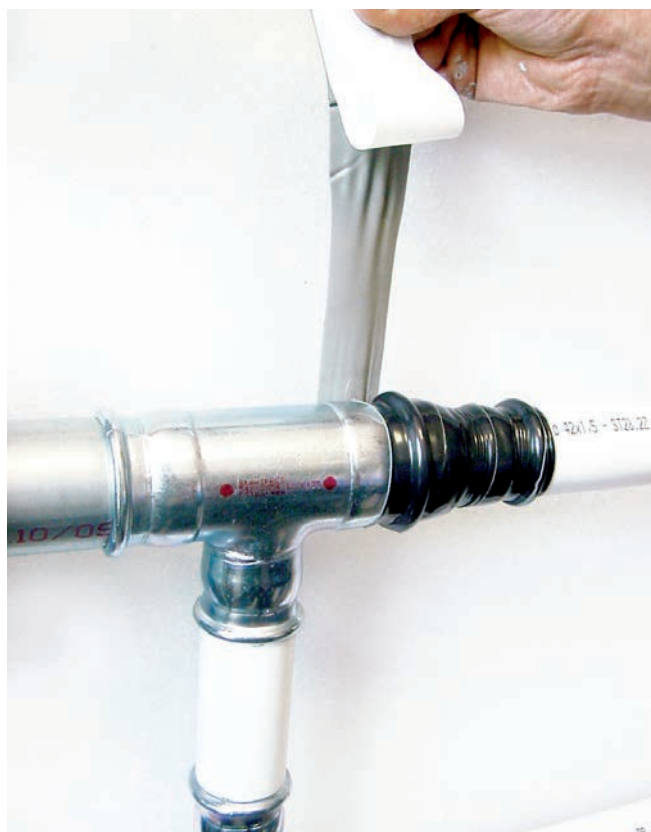
Figure 43 – Protection of the connectors with butanol adhesive tape
